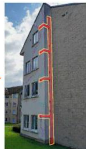
IMAGE 9 HOUSE 9, EXAMPLE OF BOXED IN F&R RISER PIPEWORK FROM BURIED DH TO ROOF LEVEL. 4No. HIJ CONNECTIONS TO BRANCH OF MAIN RISER. PIPEWORK TO PENETRATE PERIMETER WALL WITH ISOLATION VALVES ADJACENT TO NEW HIJ'S.
