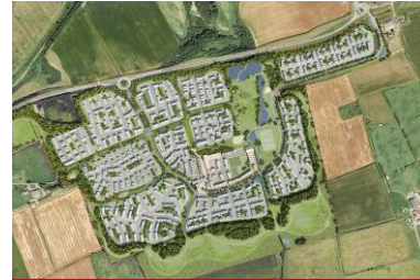
Mine Energy – South Seaham
