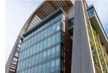
Energy from Waste - Leeds
