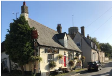
Ground Source Heat Pumps – Cambridgeshire
