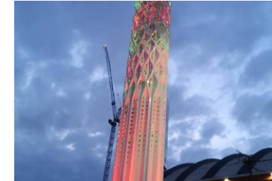
Gas CHP – Manchester
